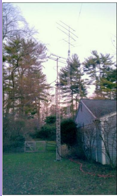
Top three antennas are loopers for 903, 1296, and 2304. The 3456 antenna that I bought from W2SJ is mounted below. Tower is a loaner from Dr. Rick. The rotator is an HD-73 that I picked up at Timonium. There is some loaner coax from K3TUF.
